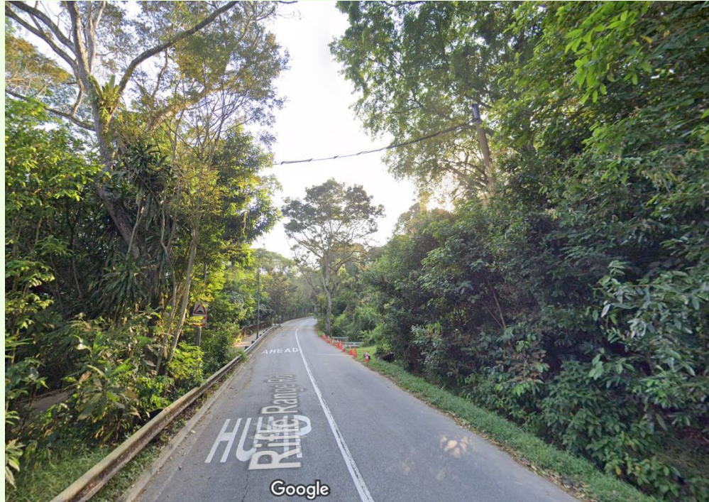
Between Visitor Pavilion and Temasek Club
