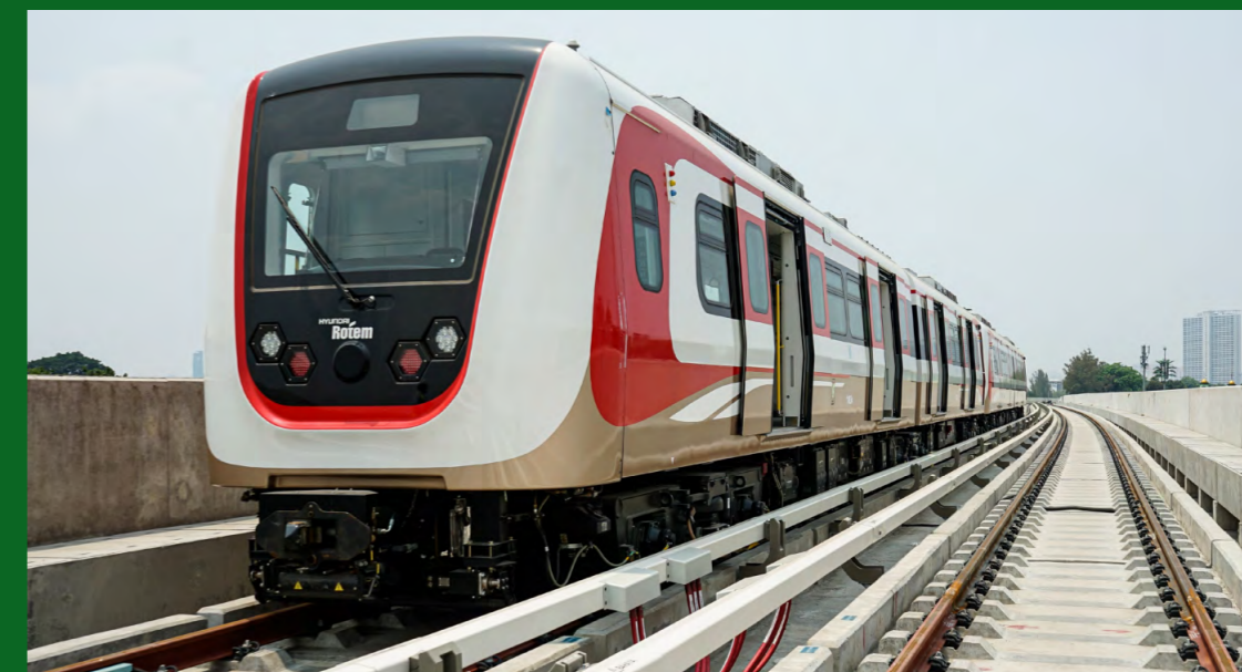
Figure 12. The Light Rail Transit Jabodebek. Source: PT SMI, 2023 81
