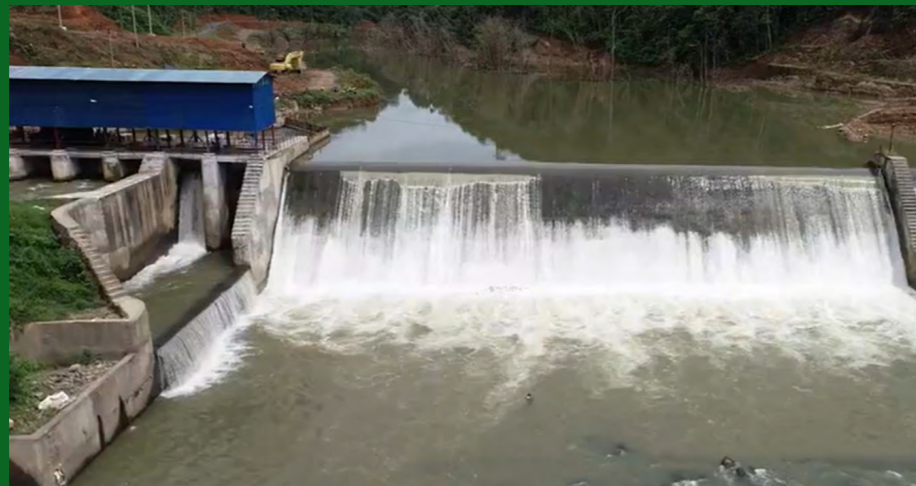
Figure 11. The Tunggang Bengkulu Mini-hydro power plant. Source: PT SMI, 2023 80
